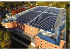
North Central College has installed 1,632 solar photovoltaic (PV) panels and energy storage system on the roof of the Residence Hall/Recreation Center (Res/Rec) that will provide 538.56 kW and 22 percent of the electricity for the building, along with immediate energy savings. The project's 12 solar inverters change the electrical current from direct to alternating current. It includes an integrated 250 kW energy storage system. The array should be operational by year's end.
